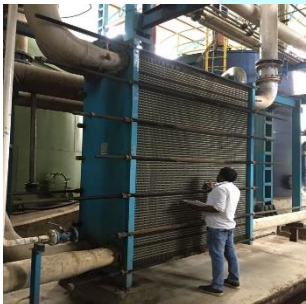
Inspection of PHE
